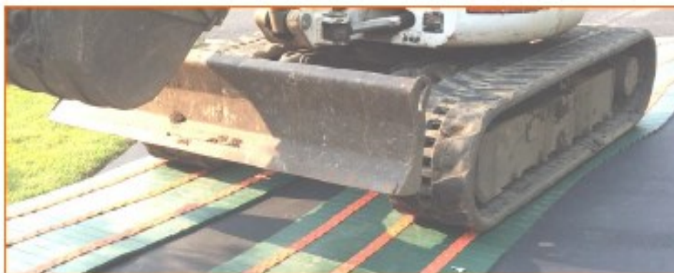
Deploy with strapping and strapping fasteners up on hardscape.
